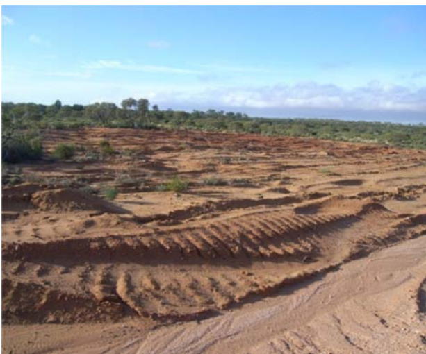
Plate 5: Pinjin Corridor Borrow pit Rehabilitation
