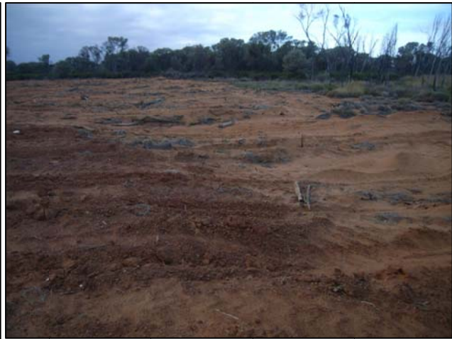
Plate 8: Pinjin Corridor Laydown Area Rehabilitation
