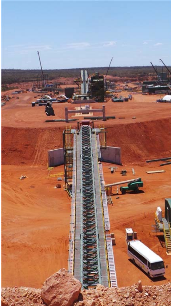
Plate 3: Conveyor Construction March 2013
