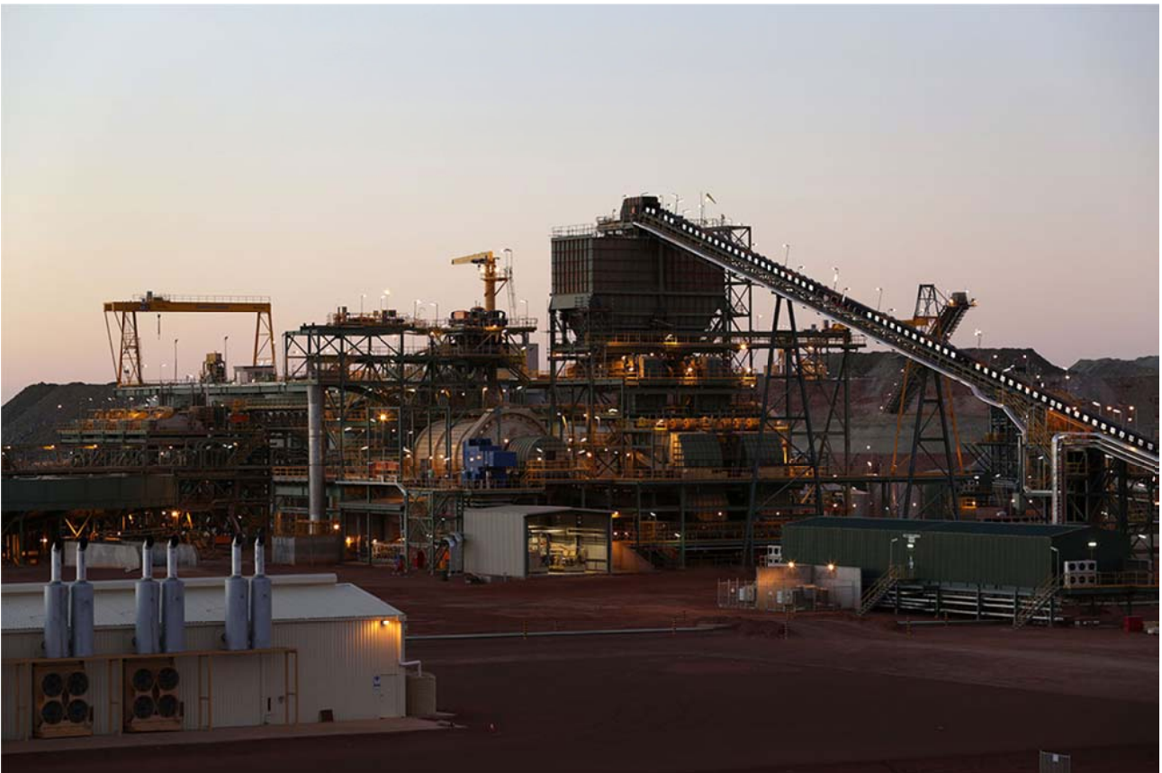
Plate 2: Processing Plant and power station September 2013
