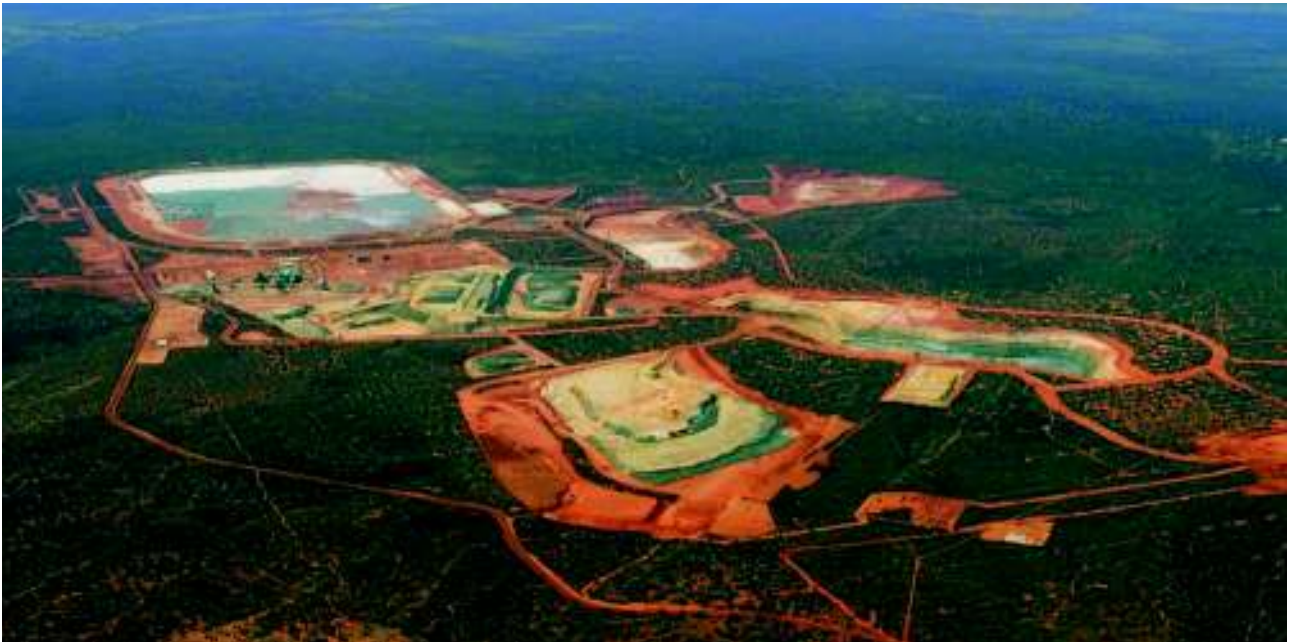
Plate 1: TGM Operational Area (October 2014 aerial) – Looking north
