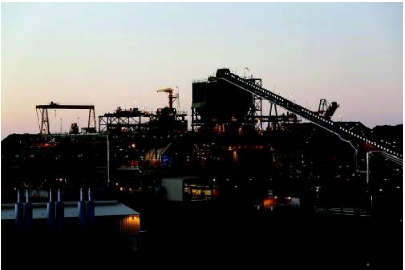
Plate 2: Processing Plant and power station September 2013
