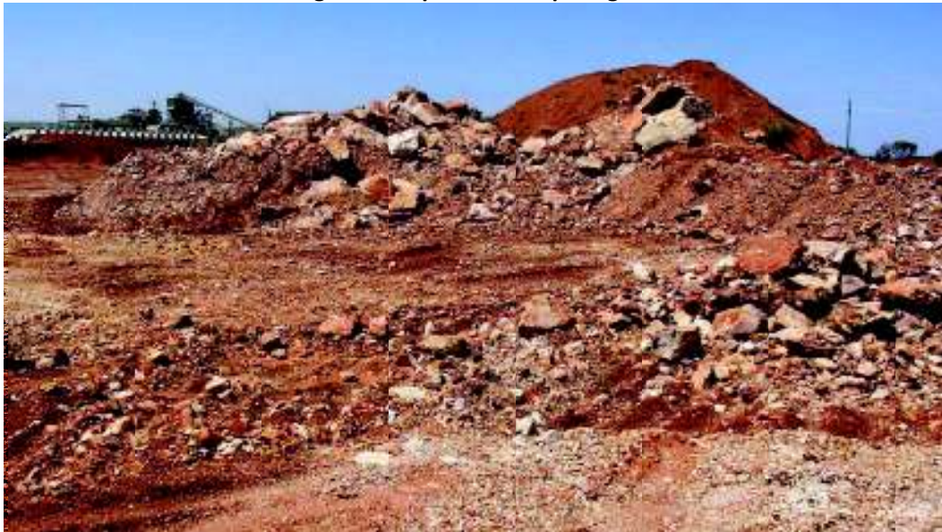
Figure 5. Pile of Calcrete to be used as Fill, for creating the 15° slope or spread across the floor of the borrow pit
