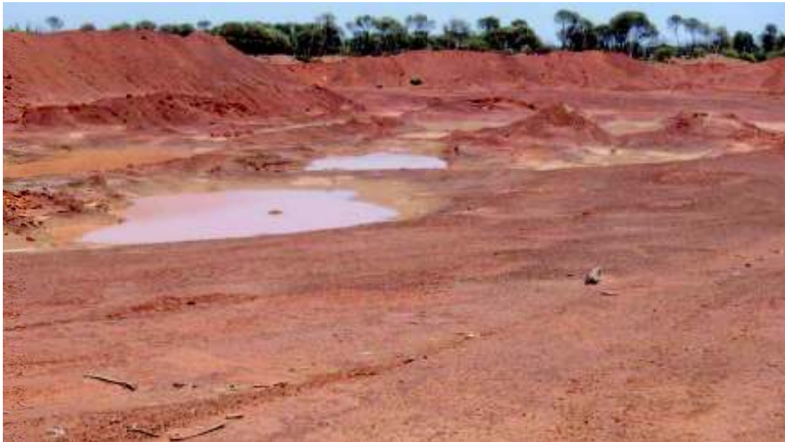
Figure 14. Depression Requiring Fill
