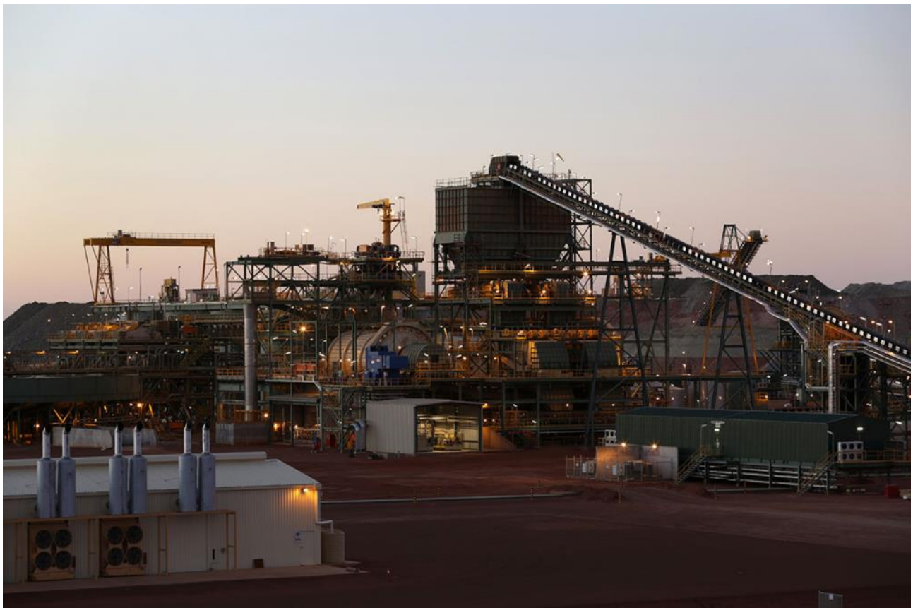
Plate 2: processing plant and power station (September 2013)
