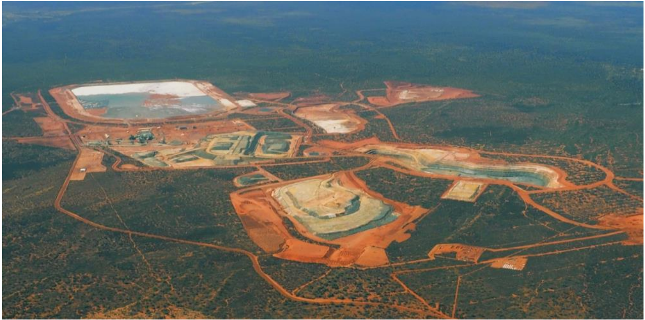
Plate 1: TGM Operational Area (October 2014 aerial) – Looking north
