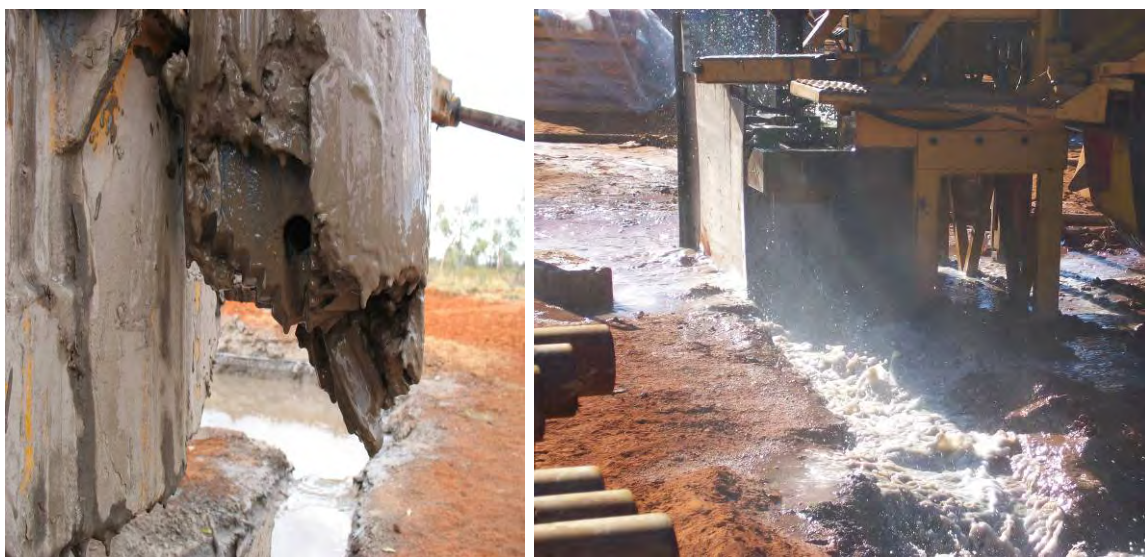
Figure 3-5: An example of a mud rotary chevron blade bit fouled by stiff grey clay (left); airlift yield in progress in the bore development phase (right).
